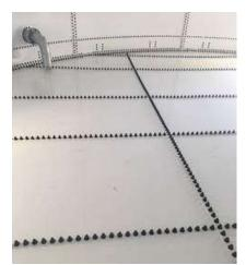
One immediate issue with using a standard flat Vacuum Box on bolted tanks is that the height of the bolts interferes with testing. To overcome this, we designed a unit with a taller profile so that the Vacuum Box can effectively encapsulate the bolts and create a successful vacuum.
